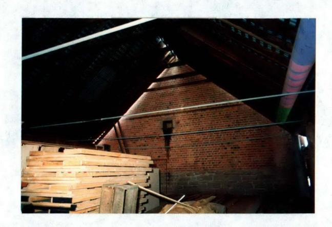
4. The rotting flooring timbers, shown in this photograph standing against the wall, were replaced by "new" floor boards.
